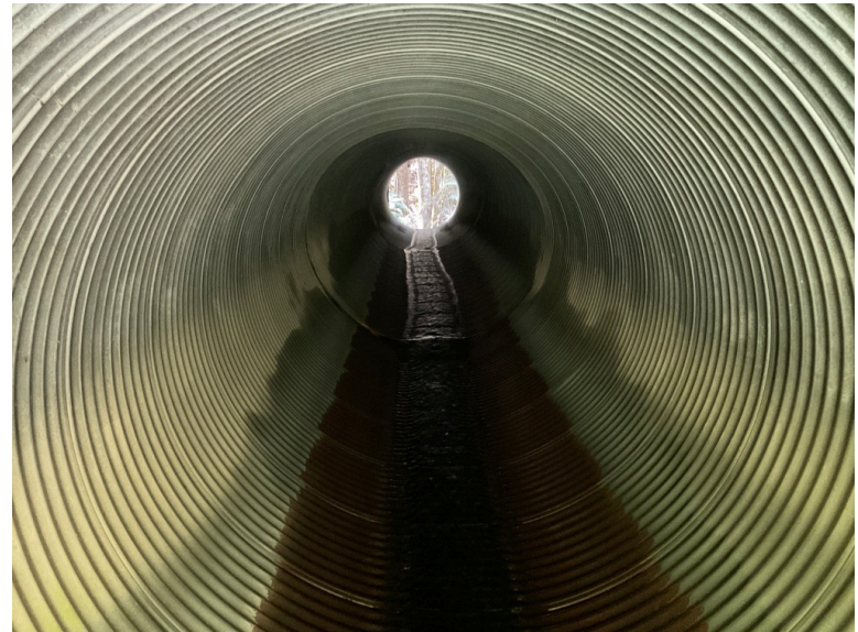
Looking Downstream Through CMP
